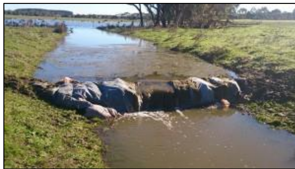
The temporary sandbag weir, operating nicely after a substantial rainfall event – notice the wetland area in the background.
