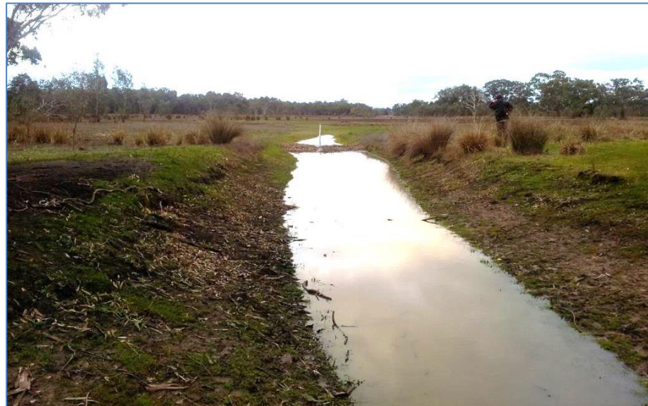
Conditions looking from the drain towards Gooseneck Swamp on the 9th August
