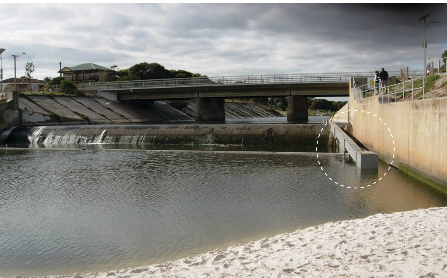
A new fish ladder (circled above) at the mouth of the River Torrens allowing movement of fish from the sea into freshwater over the Breakout Creek weir
