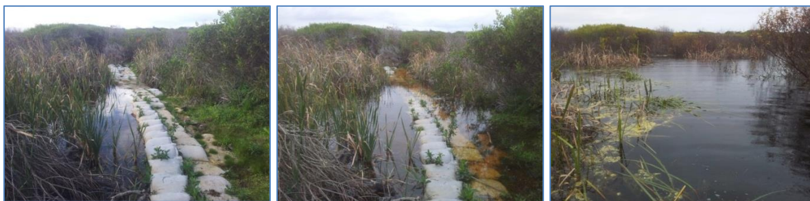
The Phase 2 structure in early April 2015 (LEFT) prior to commencement of the Phase 3 structure, in late April 2015 (CENTRE) as it became redundant for the first time, and in September 2015 (RIGHT) completely submerged as wetland levels have recovered – note the recovering aquatic reeds in the left foreground.
