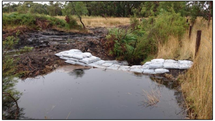
Flow Regulation Point #1: during and a short time after works were completed
