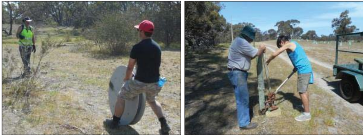
Rolling wire so it can be re-used and removing of the pine posts using large jacks (Photos by Jeanette Aslin)
