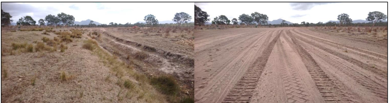
Looking west at the now completely backfilled southern outlet drain through the lunette. (Red dot on map above)
