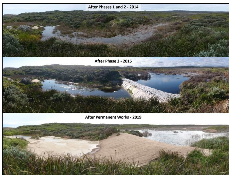
Time sequence showing the trial structure and recreated sand dune at Nobles Rocks. Photos: M. Bachmann
