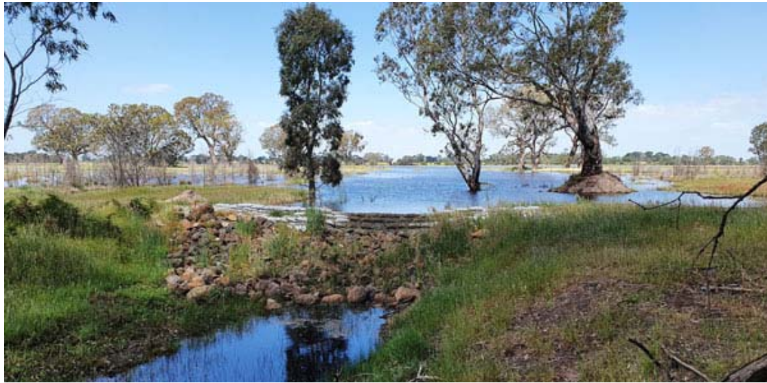
The geofabric spillway where discharge from Walker Swamp is managed back into the artificial drainage network. Shown here full with a slow trickle over the spillway on 16th November 2020. credit: Mark Bachmann.
