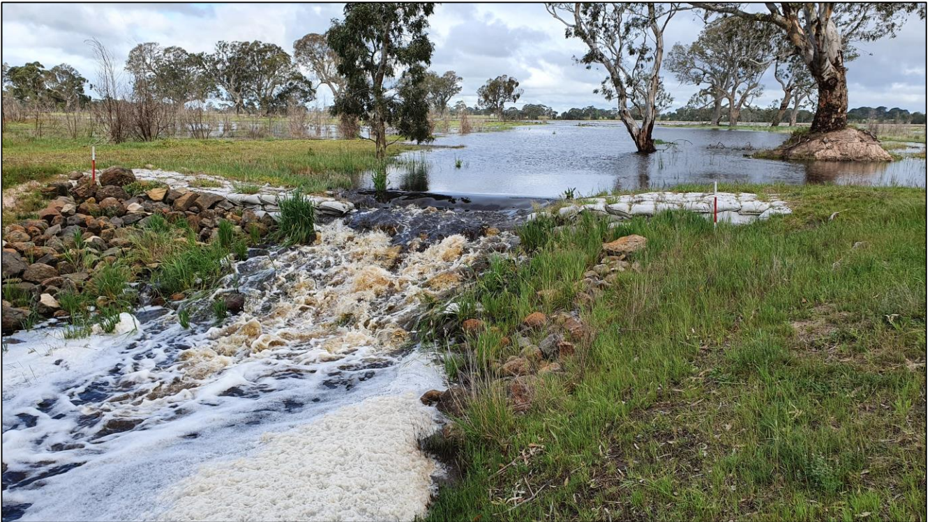
The Walker Swamp outlet spillway on the 17 th of October 2020
