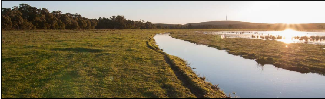
Artificial drain at Mt Burr Swamp, intercepting the perched groundwater aquifer
