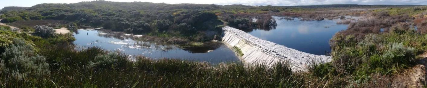
2019 - After permanent works (dune recreation)
