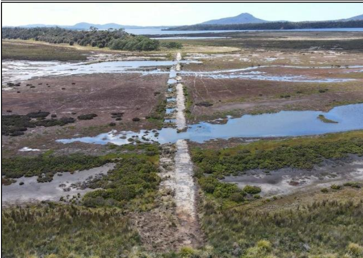
Looking north towards Long Point along the shorter (western) levee before and after the completion of remedial works in autumn 2023 (left). Right shows a close-up view of the way the spoil was arranged to prevent the channel from flowing in future and allow some saltmarsh re-establishment near natural surface.
