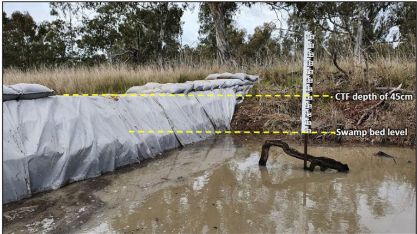
The completed restoration trial structure, showing how the channel at this location has eroded below the bed level of the swamp, and the restored CTF level. Photo: Mark Bachmann
