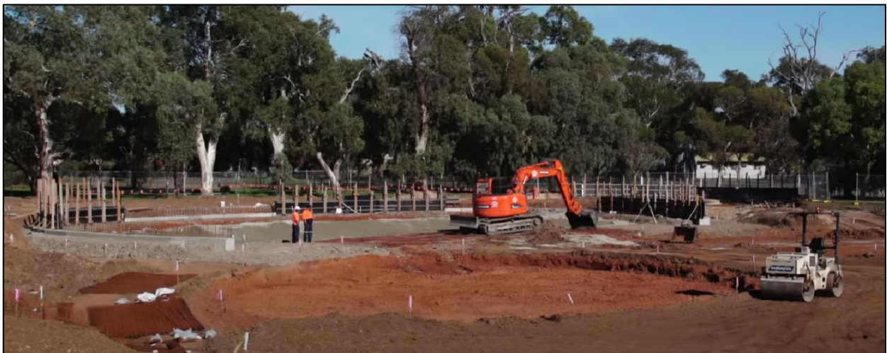
The site during construction
