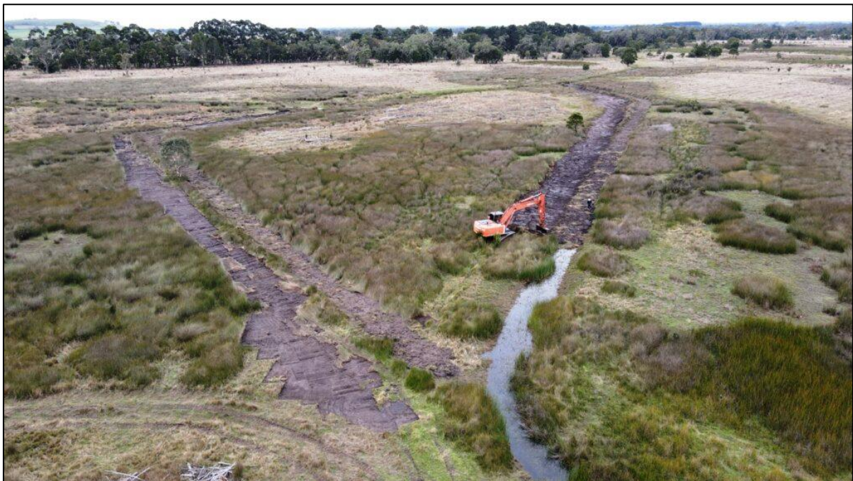
The drain backfilling process underway in the Mt Burr Swamp Stage II works area. Photo: Mark Bachmann
