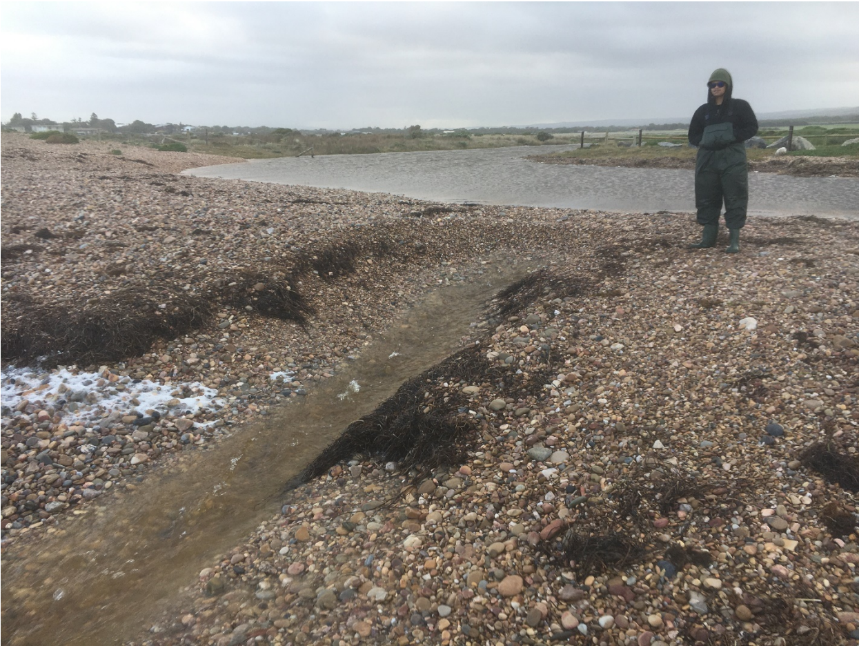
Figure 23. The Washpool outlet on 17 th July 2021, looking upstream, showing the pebble embankment in place but leaking, with water re-emerging on its beach-facing side to form a fast flowing stream. Onlooker is Drew Kilner (photo: Ben Taylor).
