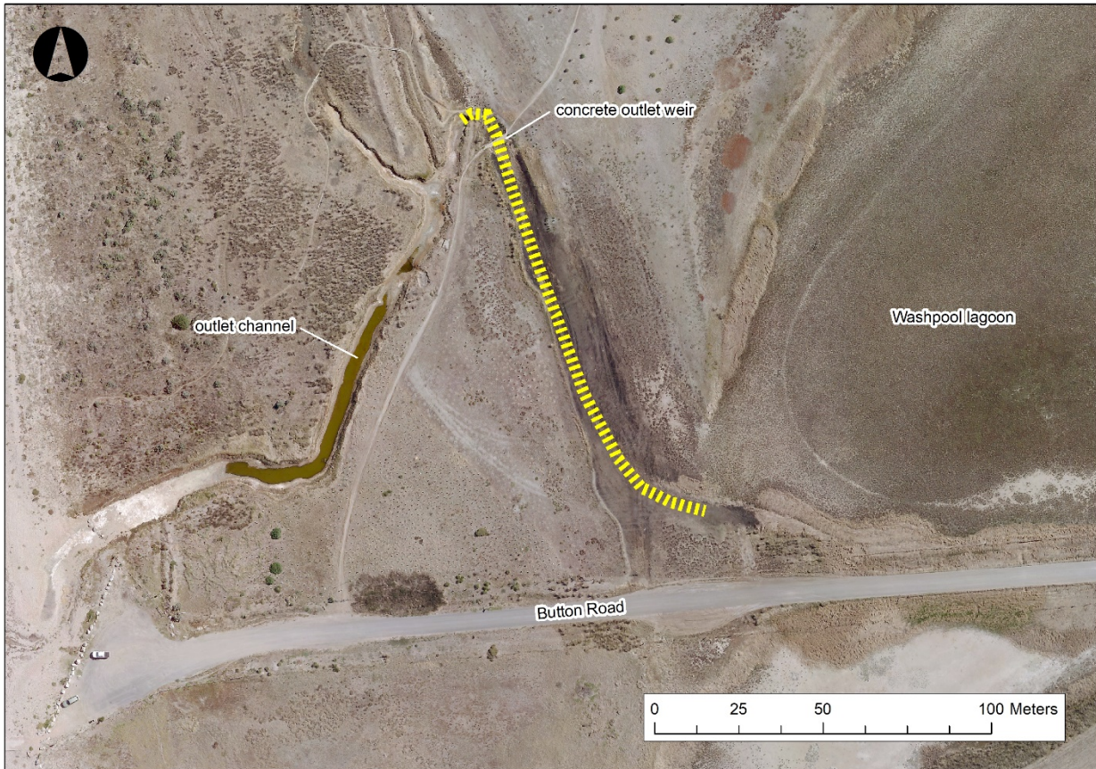
Figure 50. Existing channel (yellow dashed line) that could accommodate a rock ramp fishway at the Washpool.
