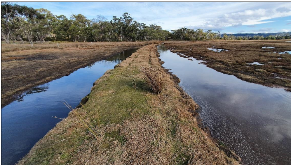
Figure 33. Looking south along the vehicle access causeway constructed c. 1990. Photo: Mark Bachmann.
