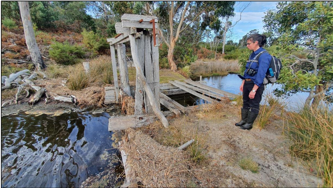
Figure 32. Close up of the timber weir constructed c. 1990. Photo: Mark Bachmann.
