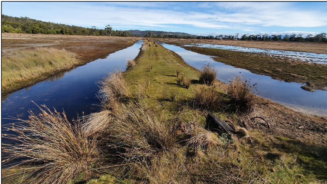
Figure 29. Vehicle causeway / crossing, with drainage channel either side, constructed c.1990. Photo: Mark Bachmann.
